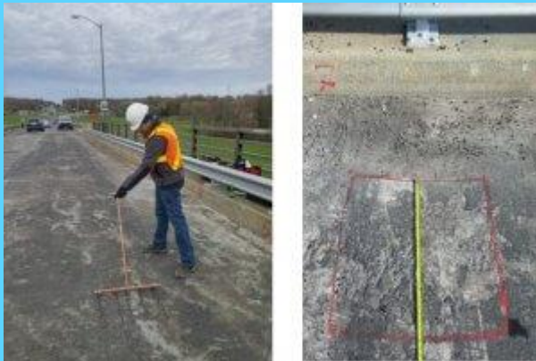
Chain Drag Delamination Survey
