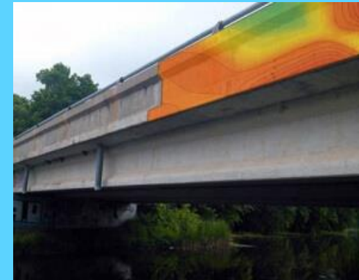
Electrical Resistivity Measurement Half-Cell Corrosion Potential Mapping
